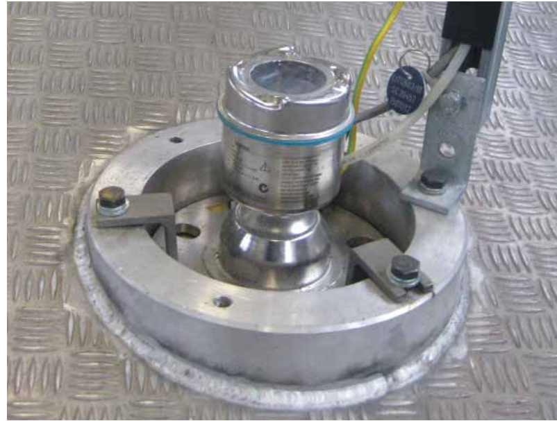
Operators easily installed SITRANS LR560 onto the fillingsilos and have seen a reduction in cleaning costs along with an increase in product quality.
